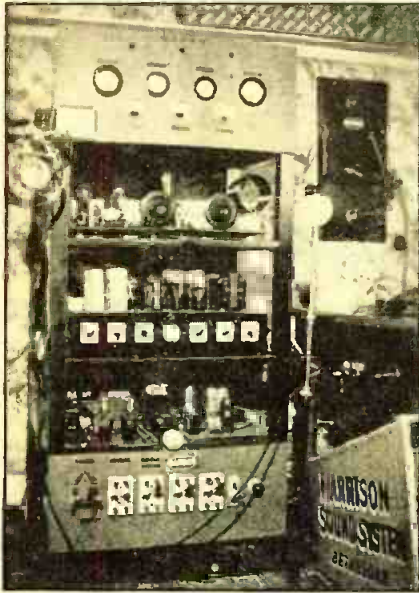
Figure 6. The P. A. amplifier is part of this amateur transmitter.
